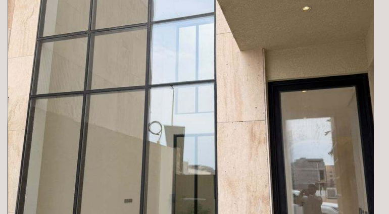
الترجيح الزاوي من الخارج CORNER GLAZING FROM OUTSIDE SOL is a trademark of Modern Distinguished Contracting Est.
