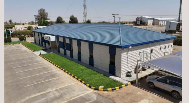
الواجهة الجانبية وسقف القرميد SIDE ELEVATION AND TILED ROOF SOL is a trademark of Modern Distinguished Contracting Est.
