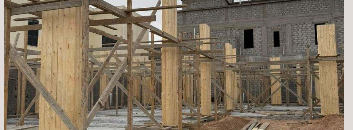
قوالب الأعمدة والدعامات الخشبية COLUMN FORMS AND TIMBER SHORING SOL is a trademark of Modern Distinguished Contracting Est.
