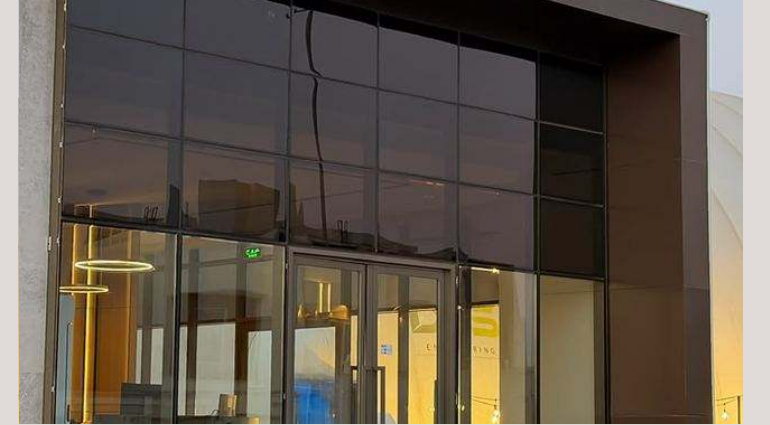
المدخل الزجاجي الرئيسي MAIN GLAZED ENTRANCE SOL is a trademark of Modern Distinguished Contracting Est.
