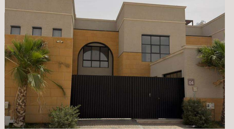
واجهة فيلا بقوس حجري VILLA FAÇADE WITH STONE ARCH SOL is a trademark of Modern Distinguished Contracting Est.
